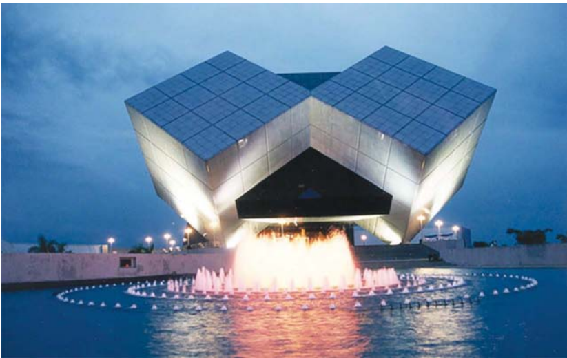
Figure 36.2: Night view of the iconic cube building of the National Science Museum, located in Pathum Thani province, 40 km north of Bangkok, which was opened to the public in 2000. The building was especially designed to present a new image of a modern science museum.
