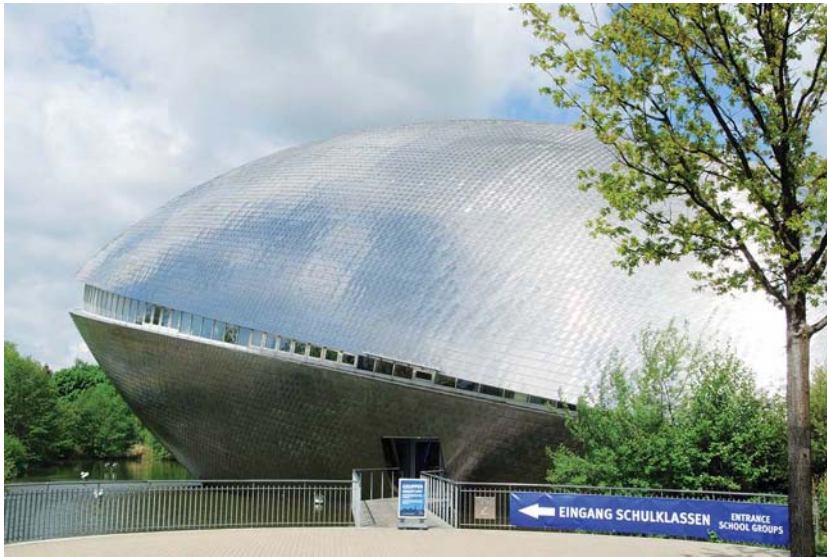
Figure 14.2: Universum Bremen, the first ‘large’ modern science centre in Germany.
