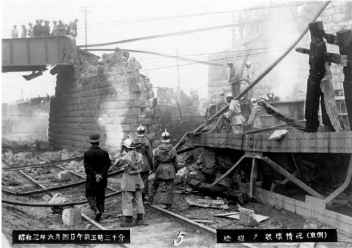
Figure 2.6. The damaged rail bridge after the bombing of Zhang Zuolin’s train just outside Mukden. The caption says in Japanese: “4 June 1928, 5:30 a.m., conditions of destruction of the bridge base (east side).”
