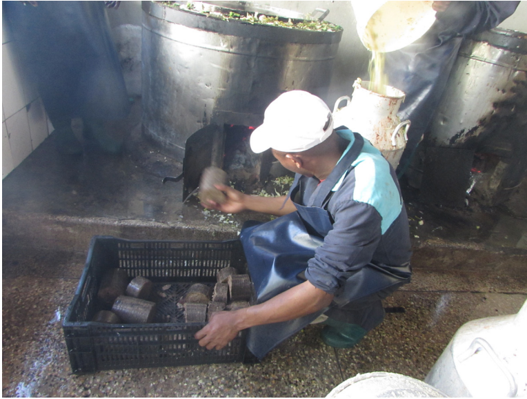
Figure 7.5 Sanivation's Superlogs being used in an industrial boiler at a flower farm in Naivasha, Kenya (image credit: Sanivation).
