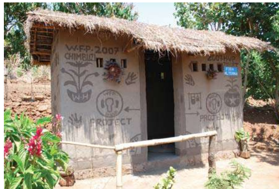
Figure 12.1 An Fossa Alterna latrine – an example of an ECOSAN latrine in Malawi.
