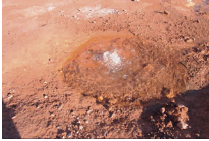
FIGURE 1.5 A CO 2 leak in Utah, USA PHOTOGRAPH BY ALVAR BRAATHEN
