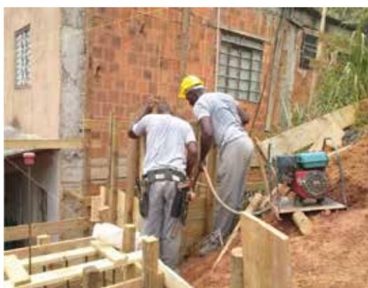
Figure 4. Vibration of concrete mix.
