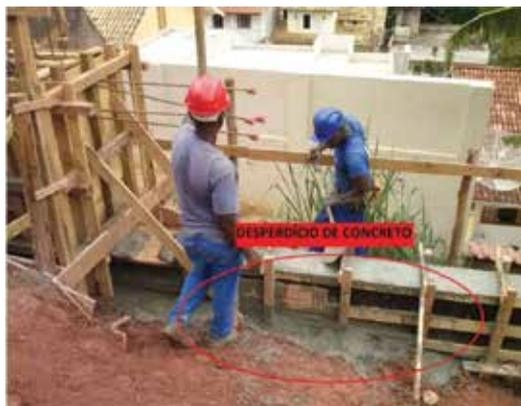
**Figure 5.** Concrete waste.
