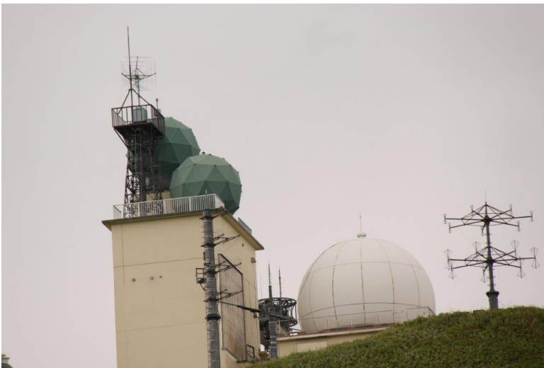
Plate 2. JGSDF Coastal Surveillance Unit 301, Maruyama, September 2011
