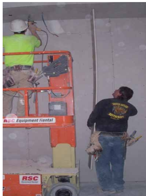
Figure 3. Use of ‘Deadman: narrow piece of panel’.
