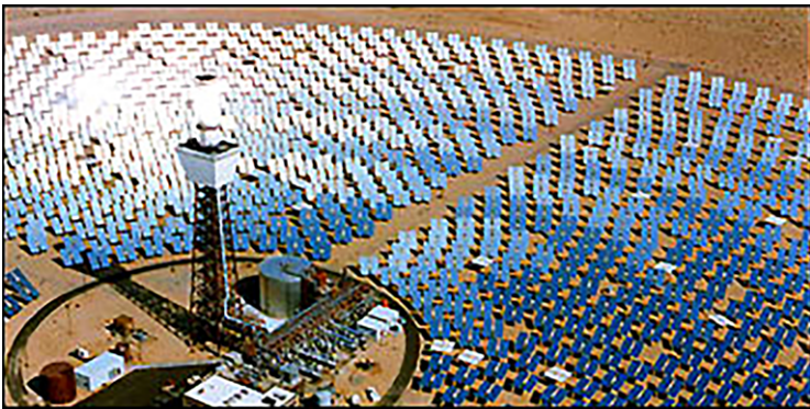
Figure 8.6 Solar One power tower plant (Source: U.S. National Renewable Energy Laboratory).
