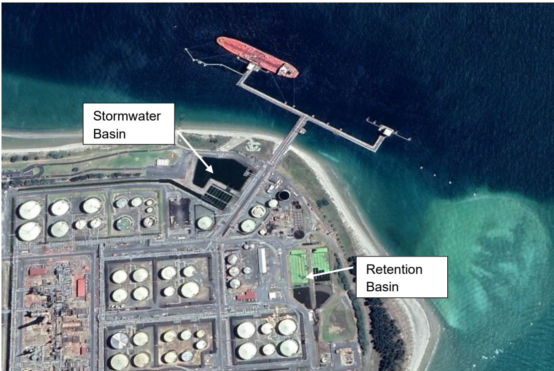
Figure 2: RNZ site showing location of the retention basin and the stormwater basin
