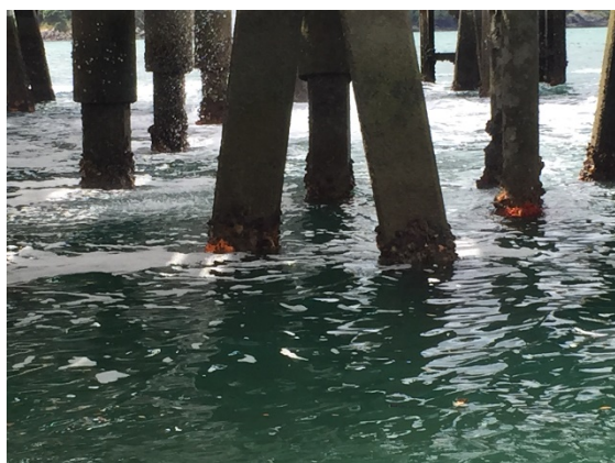
Photograph 34: Piers beneath the RNZ jetty (showing intertidal oysters attached to piers).
