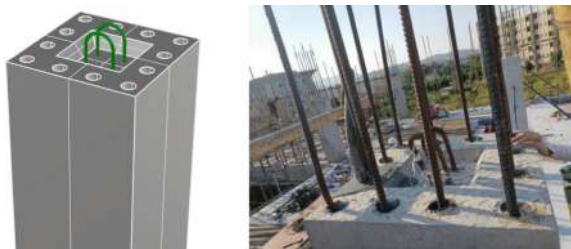
Fig. 7. Bellows through hole prefabricated column
