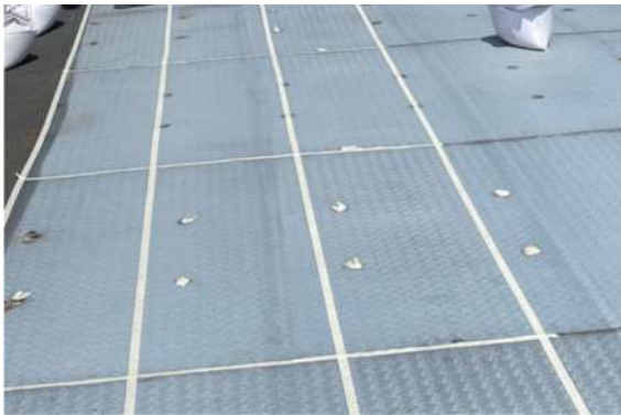
Fig. 6. Treatment of seam leaving at anchor bolt
