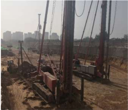
b) Compacted pile method
