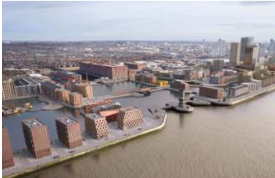
Fig. 13. Liverpool Waters Development (image: © ARUP / Peel).
