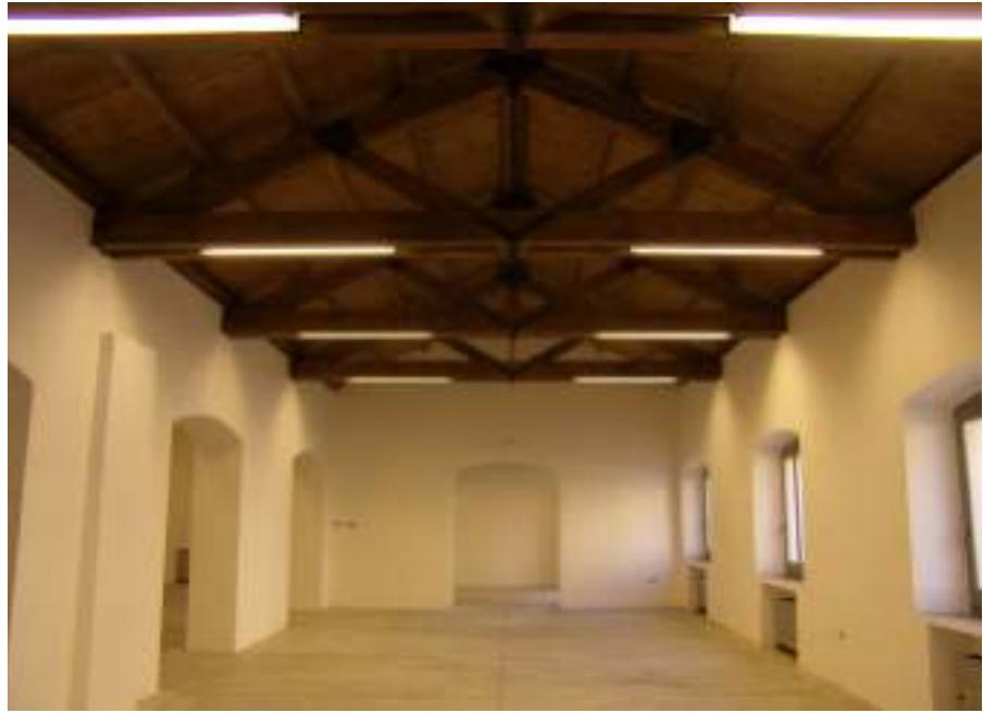
Fig. 13. Interior spaces after design and restoration work ((photograph: Pasquale Miano Studio).
