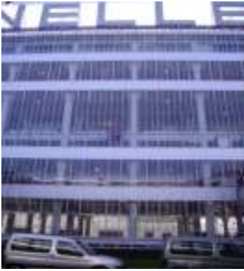
Fig. 2. Van Nelle Fabriek, Rotterdam, Johannes Andreas Brinkman, 1925-1931. Design Reuse by Wessel de Jonge 1999-2004. Facade (Paola Ascione, 2008).
