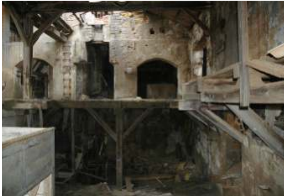
Fig. 5. The interior spaces of the abandoned machine-building (photograph: P. Miano).
