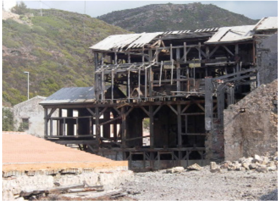
Fig. 3. The ruins of the old machine-building (photograph: P. Miano).
