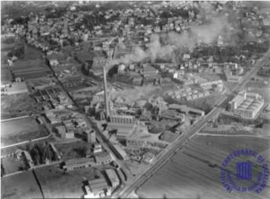
Fig. 2. Aerial view of the factory in the 1960s. Source: Cartoteca del Instituto Cartográfico de Cataluña ( http://patrimoniminerdecatalunya.blogspot.com/2014/06/fabrica-de-ciment-de-sant-just.html ).
