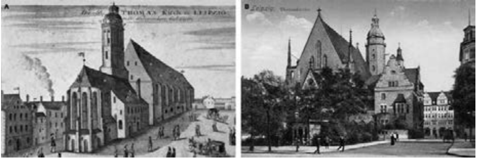
Figure 3.3. (A) A drawing of the Thomaskirche from 1749, by Joachim Ernst Scheffler. (B) A postcard image of the Thomaskirche displayed from the other side from 1918. The church's outer construction underwent a number of modifications during the nineteenth century.
