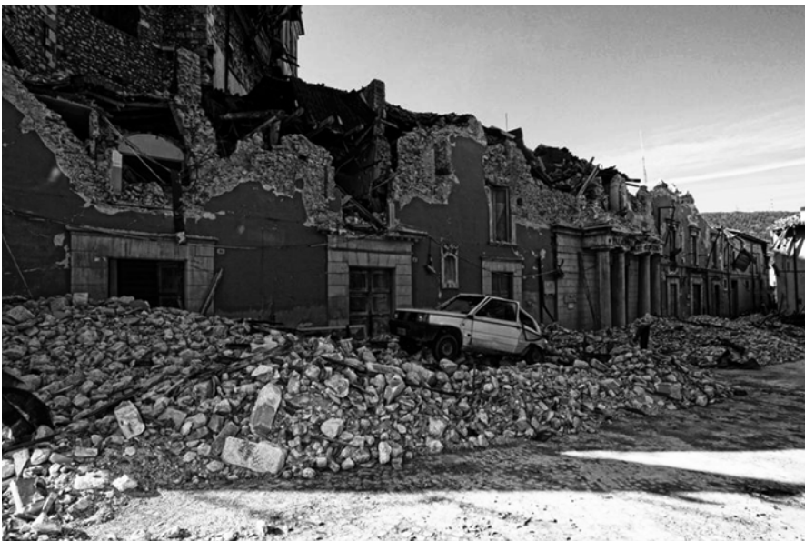
Fig. 3.6 Damage from 2009 L’Aquila Earthquake (Website of the Italian Civil Protection Department – Presidency of the Council of Ministers, http://www.protezionecivile.gov.it/jcms/en/descrizione_sismico.wp?sessionId=6EED29F25DA52C422634EE009FC67CAE?pagtab=3 )
