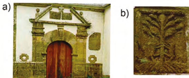
Figure 4. Details of the use of the carbonated serpentinite (Pedra de Toelo or Pedra de Moeche) in the architectural heritage of Galicia. This stone can be found in monuments and historical buildings from the Middle Ages. (a) Door lintels, and other architectonic ornaments in the façade of Labacengos church, in Moeche (16th century); (b) coat of arms of the Monastery of Oseira (oso means bear in Spanish).
