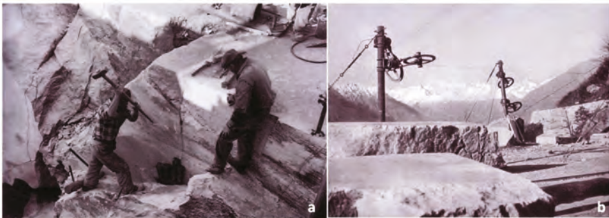
Figure 6. (a) Quarry worker with a sledgehammer, punciotti (plug and feather), and chisels. (b) Candoglia open pit yard: helicoidal wire. (Veneranda Fabbrica Historical Archive).
