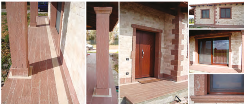
Figure 12. Some examples from a private building showing a combination of Red Montresta “trachyte” with Orosei marble (courtesy of Marmi & Pietre I.C.S. s.r.l. [15]).
