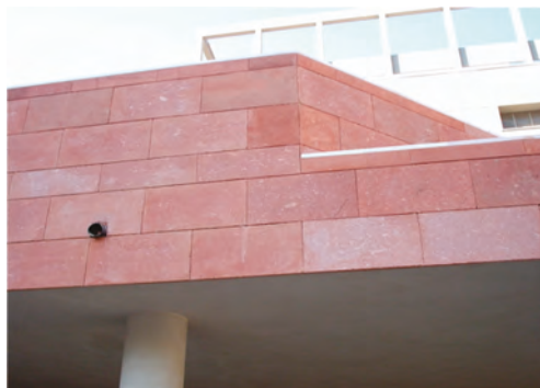
Figure 10. A detail of Teatro Massimo in Cagliari; the cladding, installed following a “run” pattern with runs in variable heights, was built using Fordongianus red “trachyte” (renewed in 2009).
