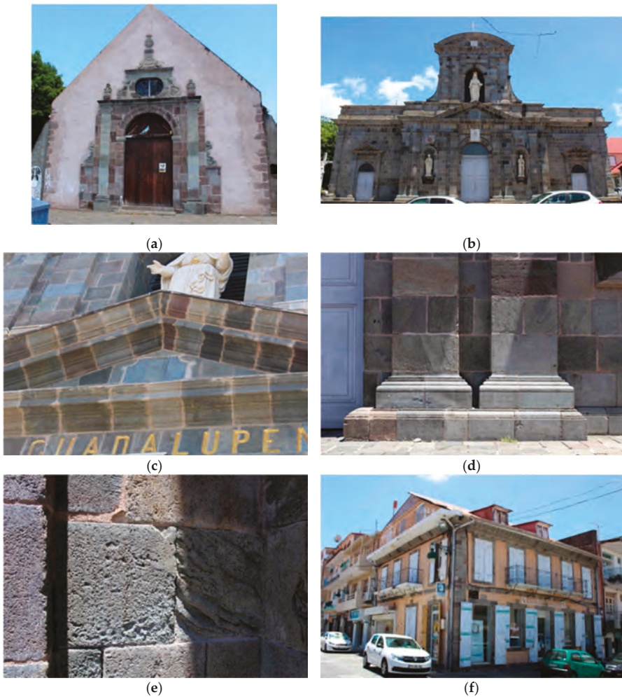
Figure 10. (a) facade of the Vieux Habitants church; (b) facade of the Basse Terre cathedral; (c) and (d) architectural elements of the Basse Terre cathedral; (e) rock alteration on the Basse Terre cathedral; (f) Basse Terre city center house, in front of the cathedral.
