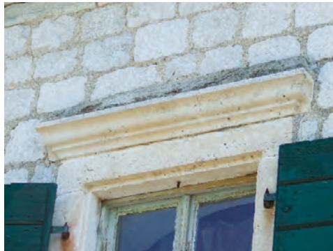
Figure 49. The frieze leans on the upper door and window frame with it's lower part (Photo: Dušan Tomanović).
