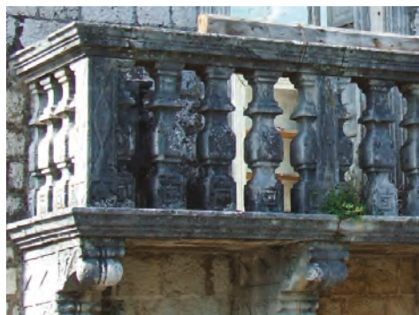
Figure 52. A type of baluster with three convex-concave parts with sharply protruding edges on the outer borders and with a square base (Photo: Dušan Tomanović).
