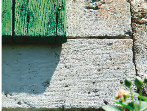
Figure 17. The Korčula stone is soft and easy to process; however, due to its lightness and brittleness, it is rarely used for construction, but only for decorating the facade (Photo: Dušan Tomanović).
