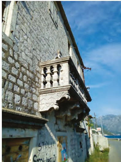
Figure 48. The regulae support heavy balconies (Photo: Dušan Tomanović).
