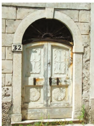
Figure 46. A stone frame above an arch-shaped door, connected by a decorative bracket at the top (Photo: Dušan Tomanović).
