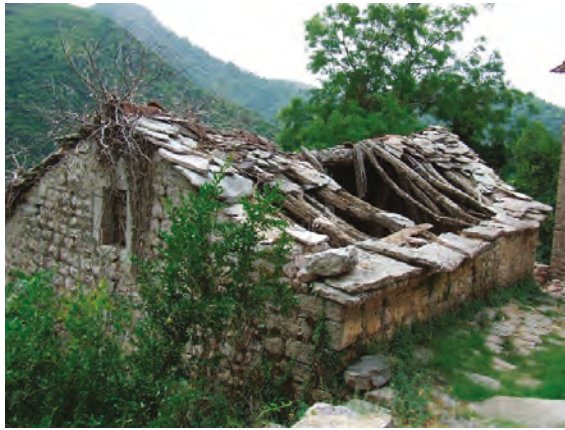
Figure 7. The single-storey stone house is at the core of rural architecture in this part of the Adriatic coast (Photo: Dušan Tomanović).
