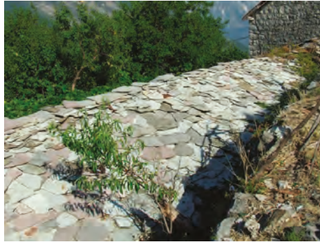
Figure 38. Flagstone roofs were dominant in the 19th century—Veće brdo (Photo: Dušan Tomanović).
