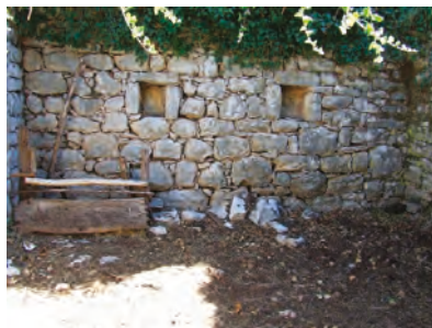
Figure 20. When present, the windows are narrow (Photo: Dušan Tomanović).
