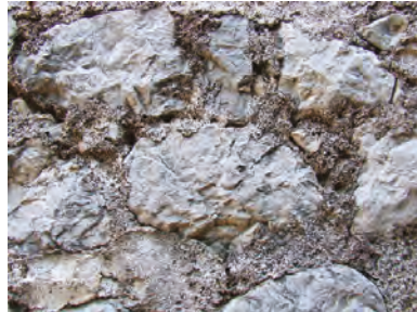
Figure 15. Less regular shaped blocks on the lateral façade from Strp and Lipci quarries (Photo: Dušan Tomanović).
