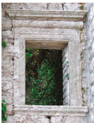
Figure 45. Frames made from Korčula stones with stylised cornices (Photo: Dušan Tomanović).
