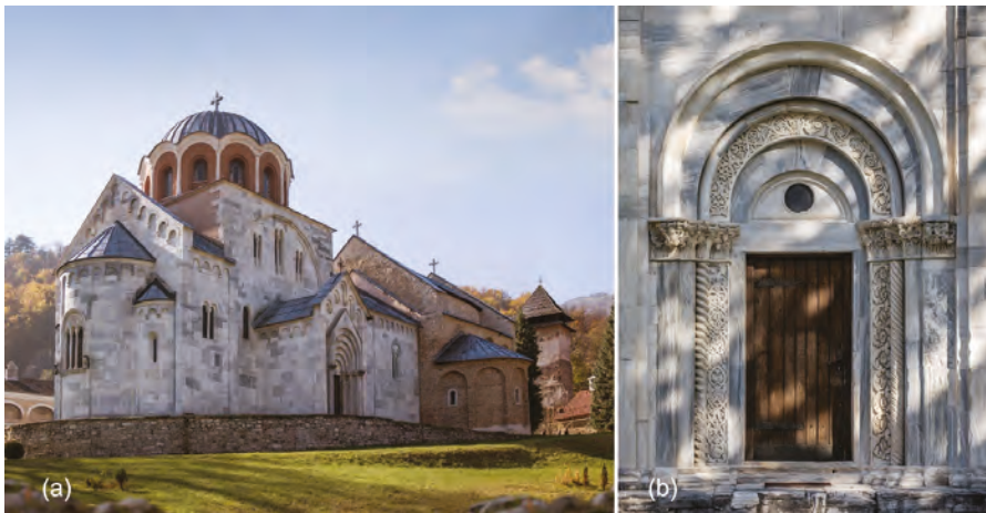
Figure 4. (a) The Church of the Holy Virgin 12th century view from the northeastern side. (b) Southern portal © LiveViewStudio.
