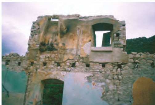
Figure 29. The floor joist beams are put into previously prepared holes in massive stone walls (Photo: Dušan Tomanović).
