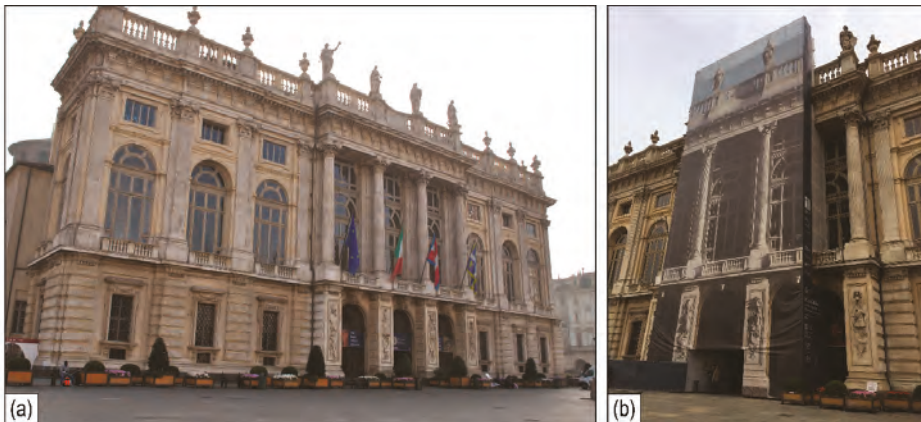
Figure 1. Buildings: (a) View of the Palazzo Madama façade; (b) Study site located in the central area of the façade.
