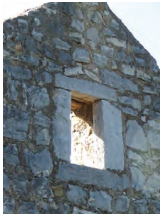
Figure 44. Window and door frames in the hinterland are mainly composed of monolithic stone with no stylised cornice (Photo: Dušan Tomanović).
