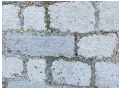
Figure 16. Front façade walls were built using the highly regarded fine stone from Strp and Lipci quarries (Photo: Dušan Tomanović).
