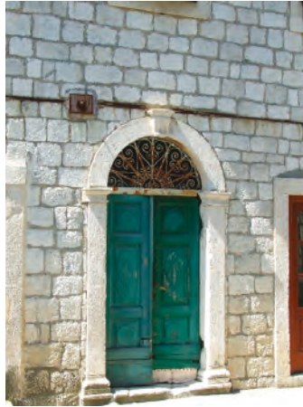
Figure 35. A door that does have fanlights is framed with arched stone frames (Photo: Dušan Tomanović).
