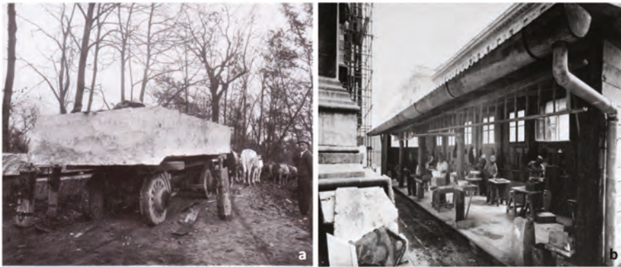
Figure 9. (a) Wagons towed by pairs of oxen which transported the blocks from the valley to the river pier. (b) Veneranda Fabbrica working yard in Milan (XIX–XX cent.) [29].
