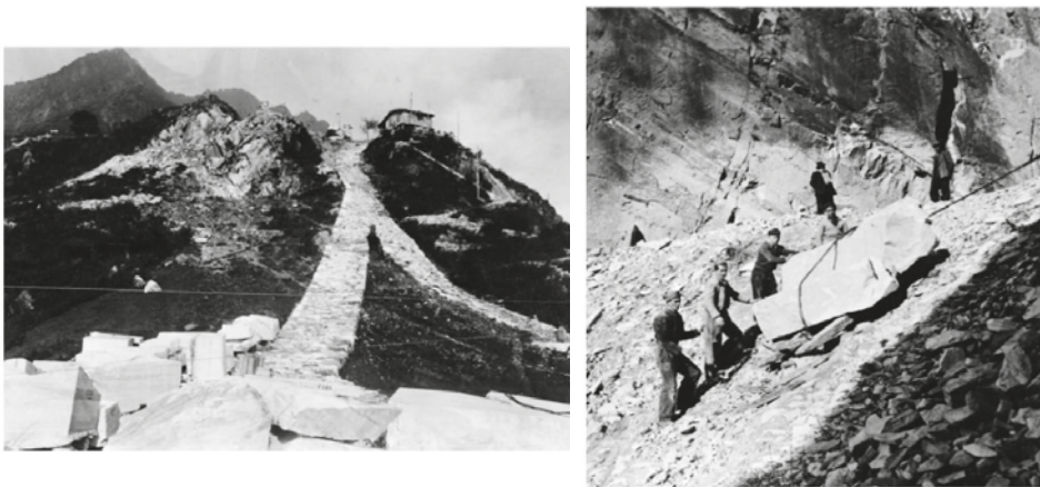
Figure 8. Running routes made of quarry waste (left) and big wooden sledges—“struse”—to transport the blocks from the quarry to the valley [29].
