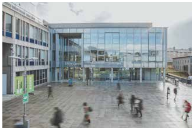
Figure 4. The STEM Centre is the University's new £18 million facility in the heart of the Colchester campus. Image © University of Essex.
