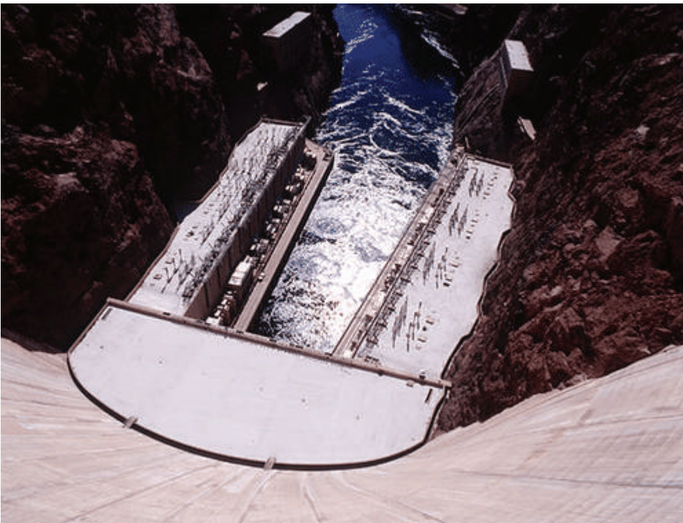
Figure 1. Hoover Power Plant View of Hoover Power Plant on the Colorado River as seen from above. Source: U.S. Department of the Interior
