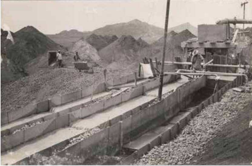
Separating tin oxide at a mine on the Jos plateau. Date unknown. Photograph by Edward Harland Duckworth. Courtesy of Northwestern University Libraries.
