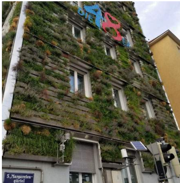
Fig. 1 “Climate façade” on the MA48 building, Vienna
