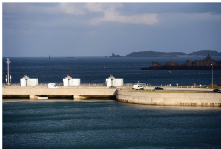
Figure 9.7: The La Rance barrage in France.
