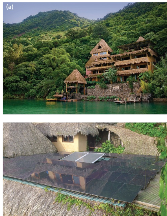
Figure 9.45: (a) The Laguna Lodge in the Tzantizotz nature reserve, Guatemala, is built from local materials, including walls made from adobe and clay and lampshades from corn paper. (b) It is a zero-carbon resort, with electricity for lighting, hot water and wifi generated by 180 solar panels.
