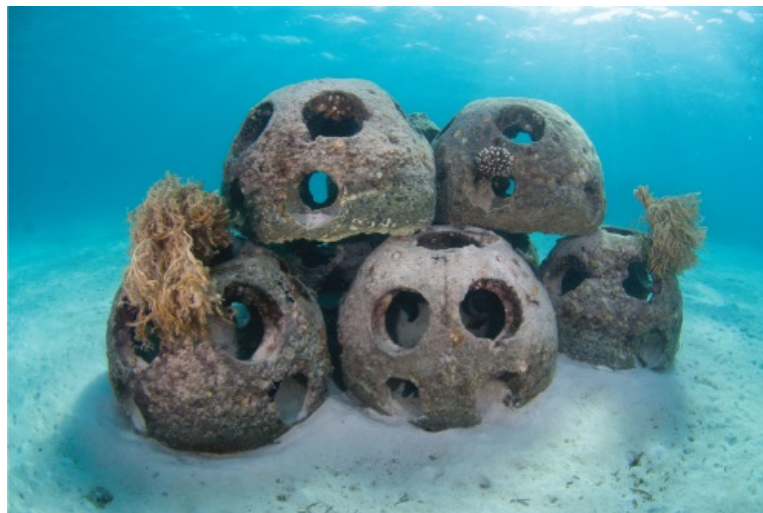
Figure 5.16: Reef balls with implanted corals placed on the soft seabed to form an artificial reef in the Maldives.
